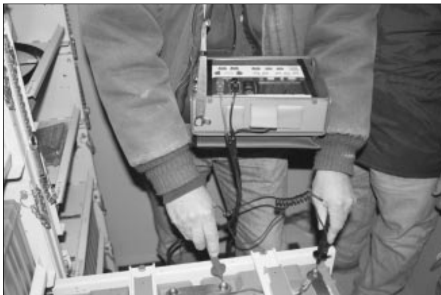
Using the C-BITE to measure 4V batteries in a CEV.
